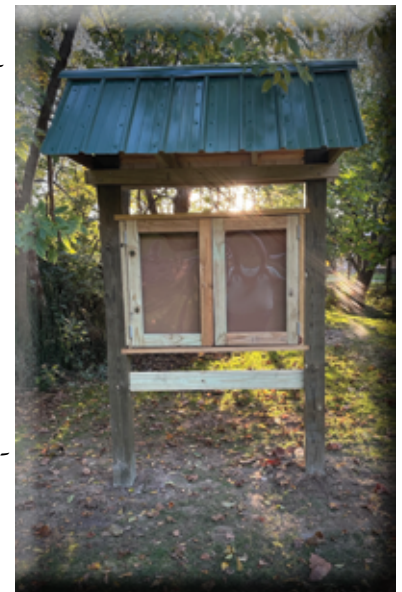
Jacob Early and crew installed this Kiosk near the entrance to Eagles Way Trail in Little Hunting Creek Park.
